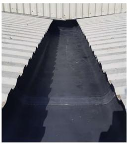
**Fixing and jointing:** Rooflock Eighteen liner is to be fixed along its length with Rooflock Aluminium trims, fixed at 200mm centres using Fastec stainless fixings. Joints formed between Rooflock Eighteen membrane liner sections to be made by Rooflock Eighteen No-Weld strip across the joint.
